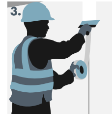
Embedding Knauf Aquapanel Exterior Joint Tape.
