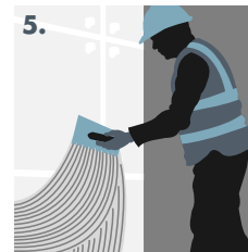
Applying notches within basecoat.
