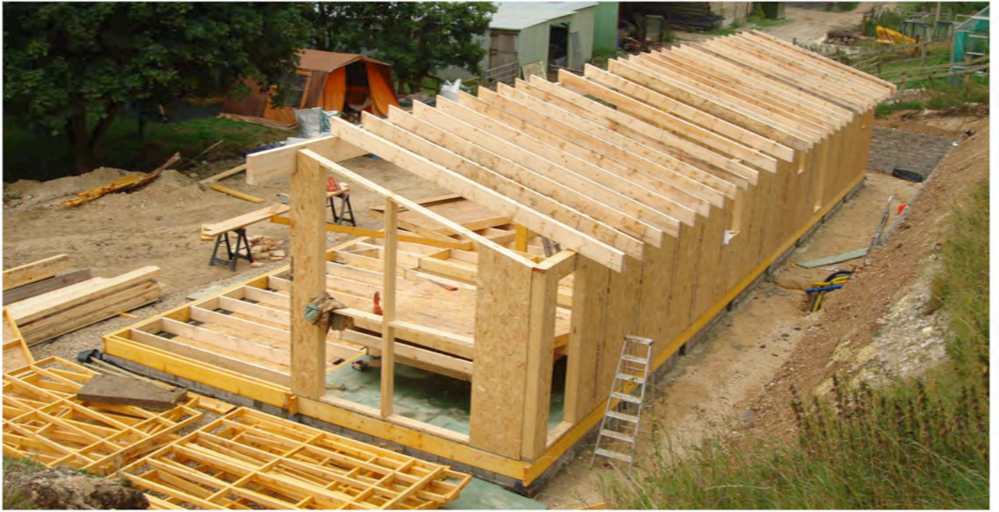
Before: Timber Frame Assembly
